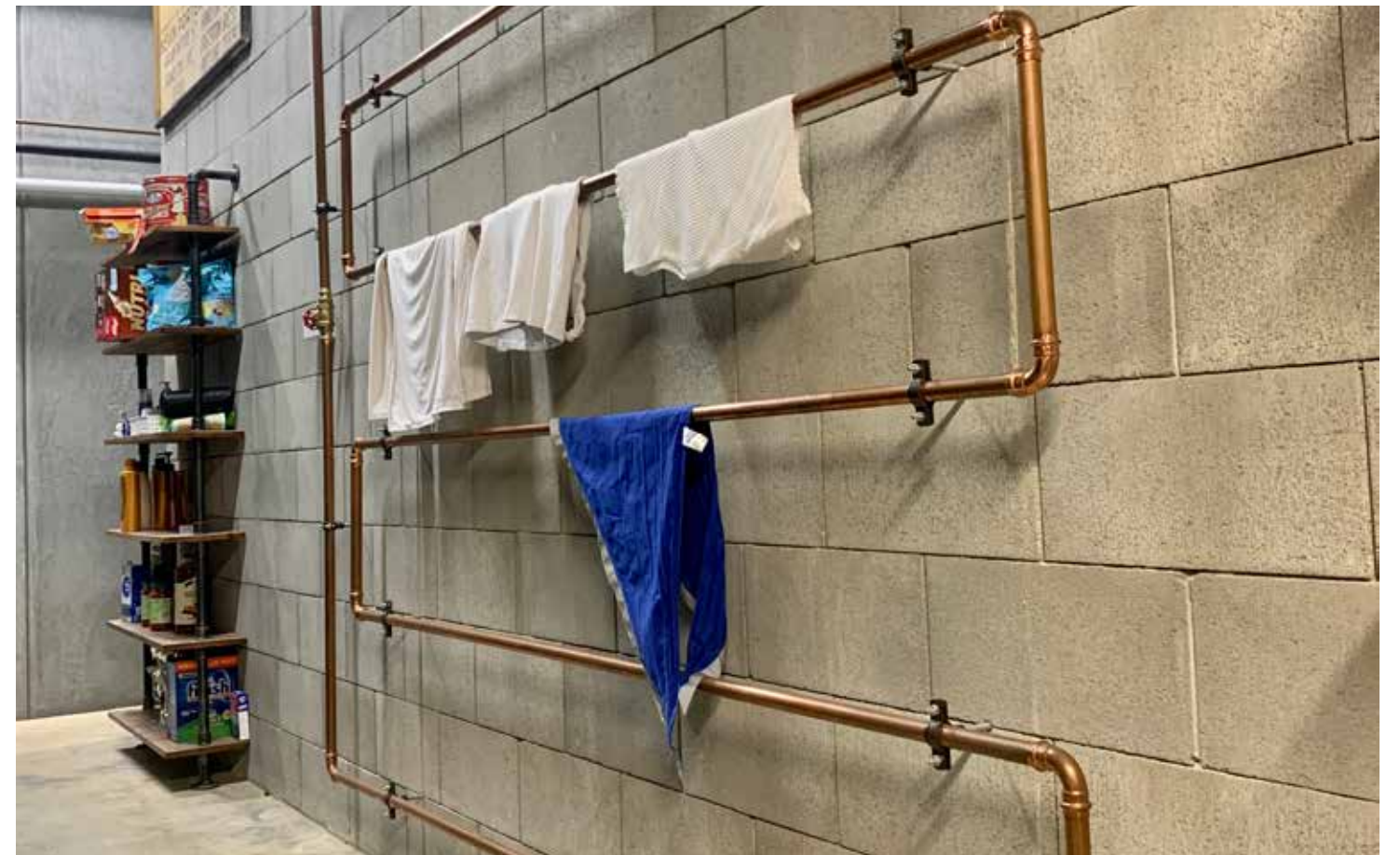
Heated clothing rack using return water from hydronic heating
