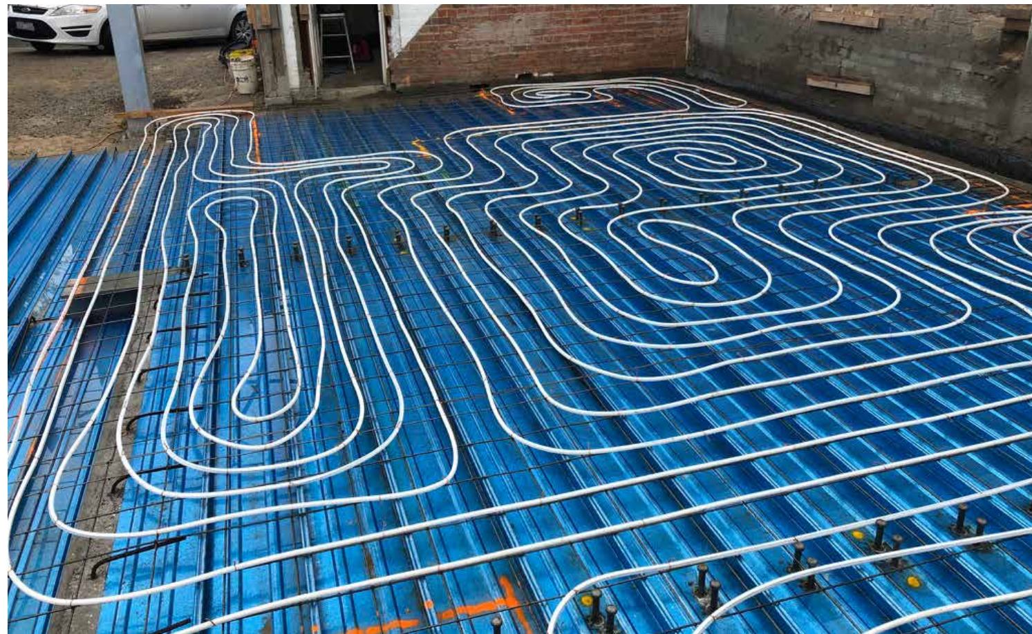
Hydronic slab heating
